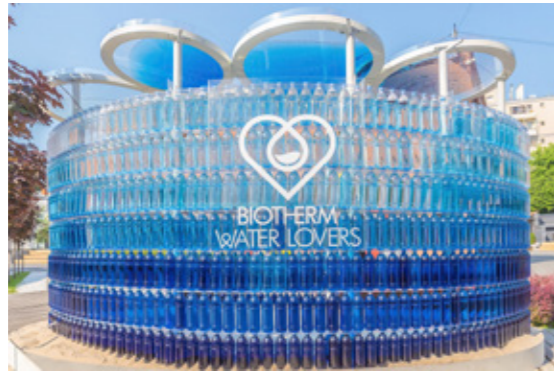
The WaterLovers pavilion Concept & design by Victor Polyakov Technical director and producer: Alexander Funtov victorpolyakov.com @_victorpolyakov_
